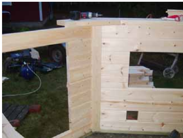
13. Fasten the inside corner fillet
