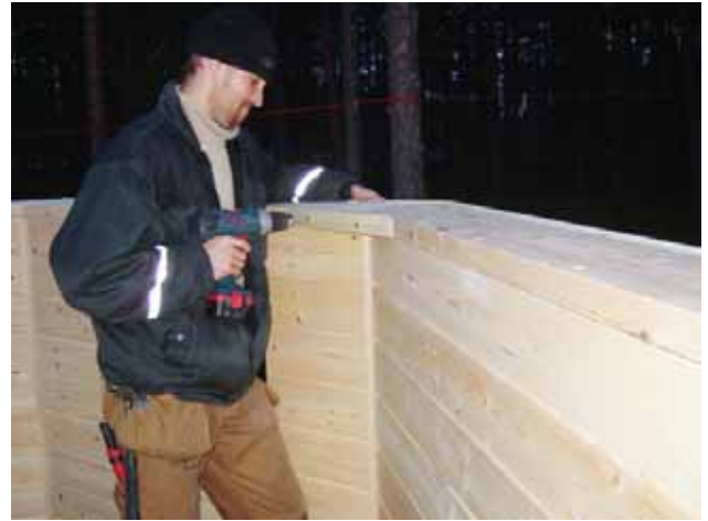
12. Attach the re-entrant corners (6 x 80).
