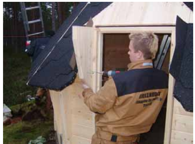
38. Put the door casing in place (6 x 80).
