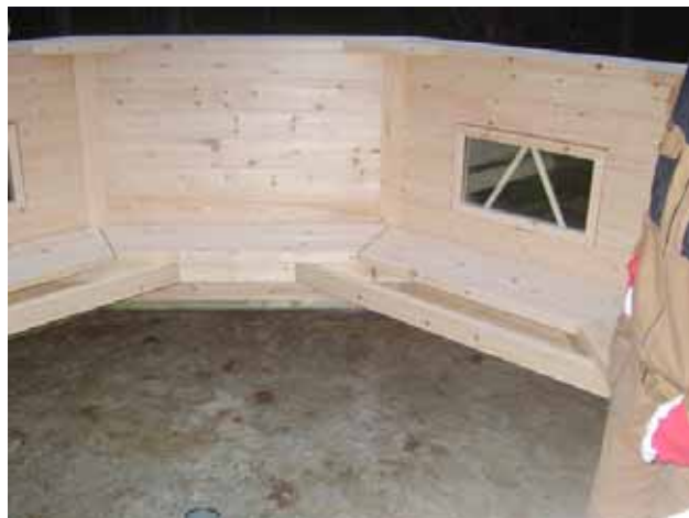
21. Put the bench planks in place.
