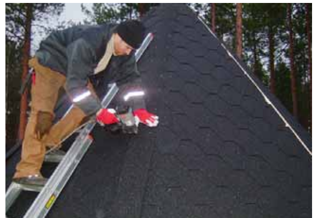
32. Fasten the composition roofing material to the corners.
