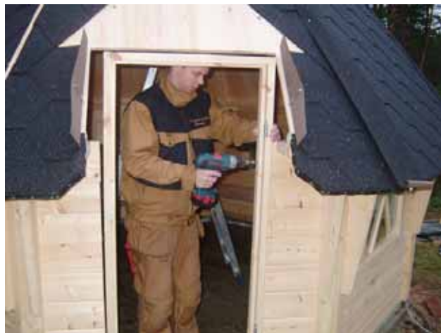
37. Fasten the doorframe so that it is even with the inside edge (6 x 110).
