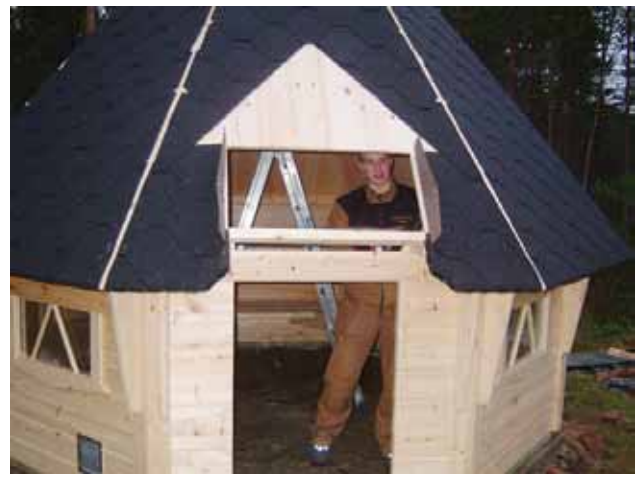
34. Saw open the door opening.
