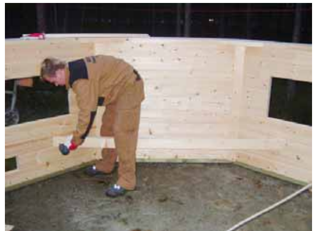
16. Fasten the three longest supports (6 x 80) first.
