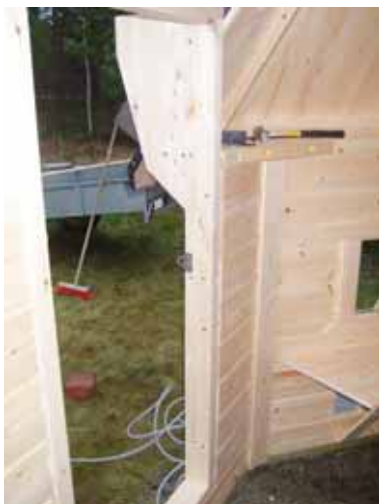
37. Fasten the doorframe so that it is even with the inside edge (6 x 110).
