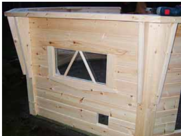
23. Install the windows and fasten the molding.
