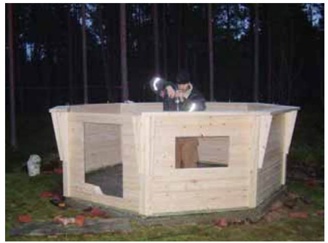
10. The short boards for the door part come last.
