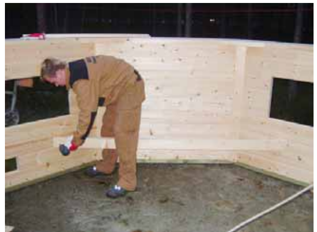
16. Fasten the three longest supports (6 x 80) first.
