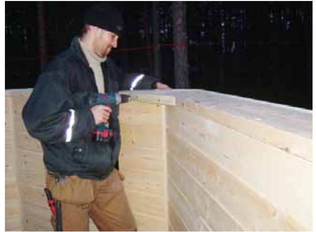
12. Attach the re-entrant corners (6 x 80).
