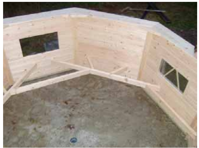
18. Fasten two supports equivalent in length to the back of the hut on the right- and left-hand sides.
