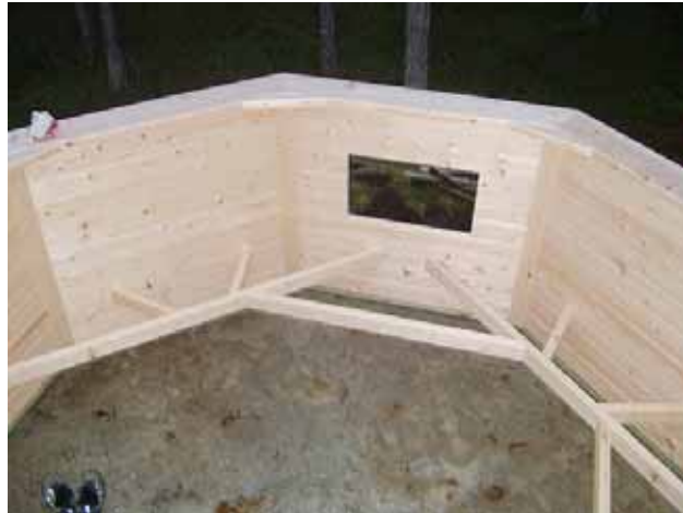
19. One support (6 x 80) goes on the right as seen from the door.
