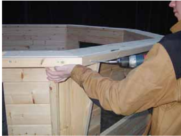
11. Screw the boards together from the outer corners (6 x 120).
