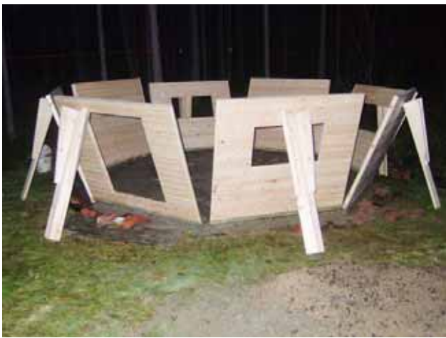
1. Put the wall elements in place.
