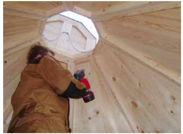
50. Fasten the chimney in place (6 x 80).
