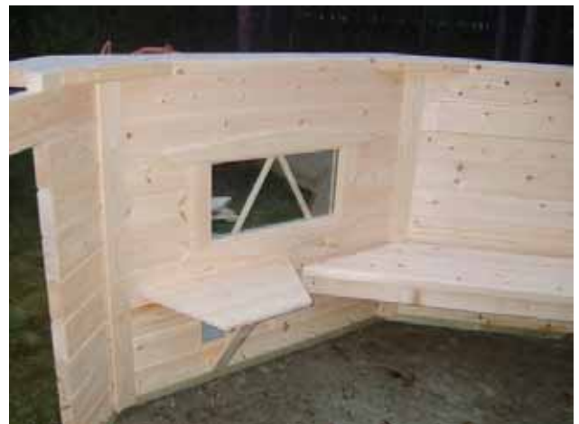
24. Fasten the side table on the wall next to the door (5 x 30).
