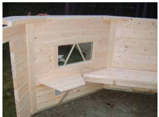
24. Fasten the side table on the wall next to the door (5 x 30).
