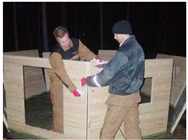
2. Attach the wall elements to each other with 6 x 120 screws.
