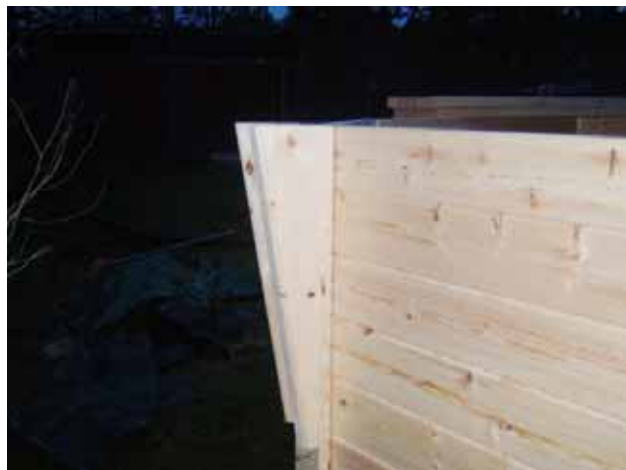
7. The upper edge should be even with the top of the wall.
