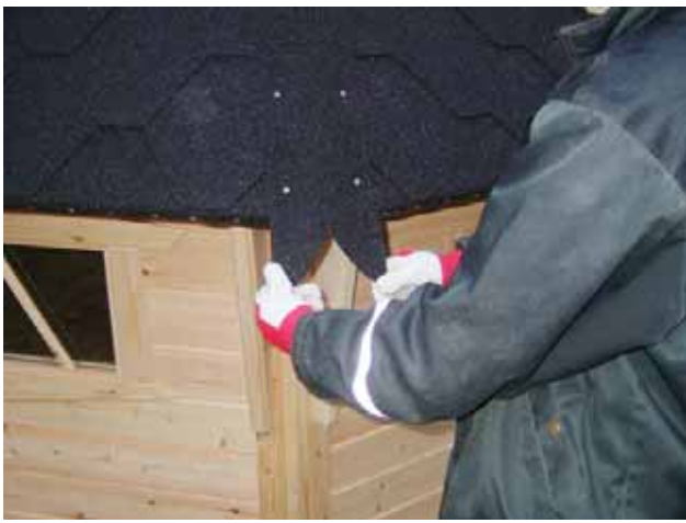
33. Cut and turn the bottom of the corners under the roof.
