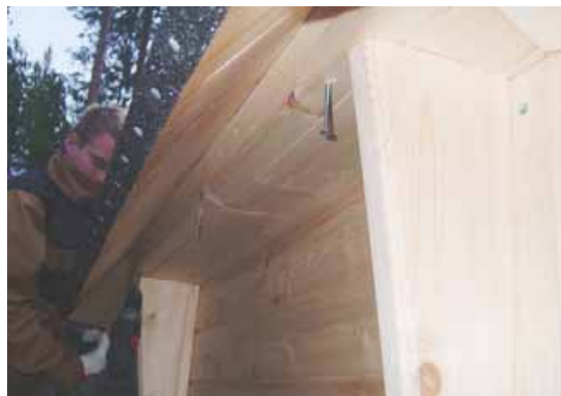
31. Fasten the roof elements to the ledges from the bottom (6 x 80).
