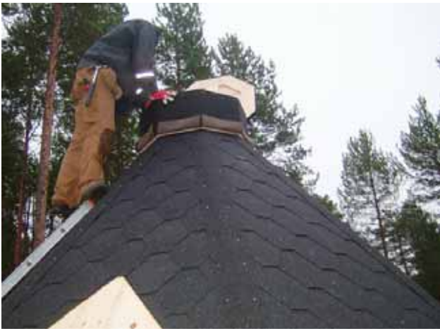
49. Put the chimney in place.
