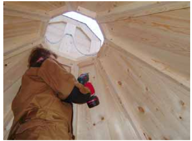
50. Fasten the chimney in place (6 x 80).
