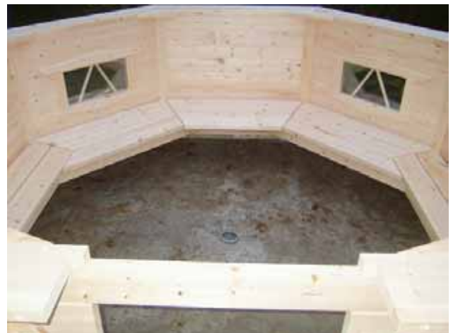
22. Fasten the bench planks (6 x 80).
