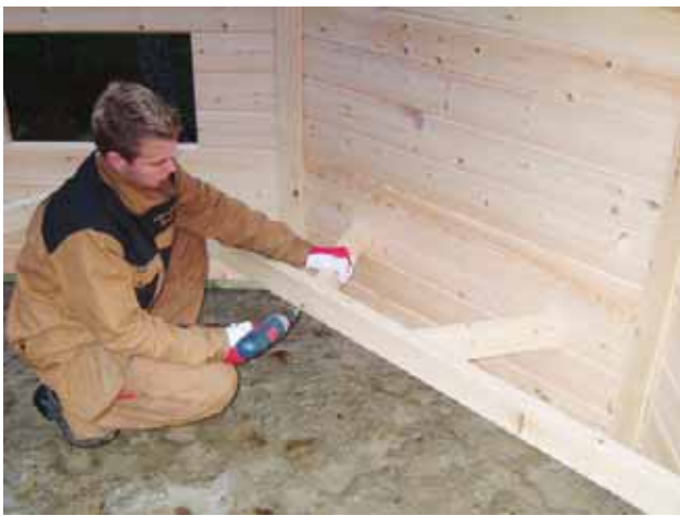
17. Then install the six shortest supports (6 x 80).
