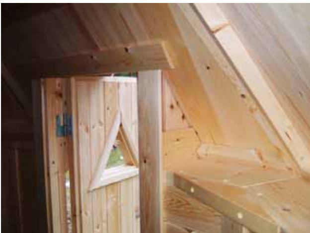
47. Fasten the door molding inside and outside.
