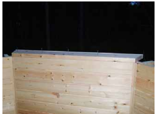
8. Fasten the ledges on top of the wall (6 x 80).
