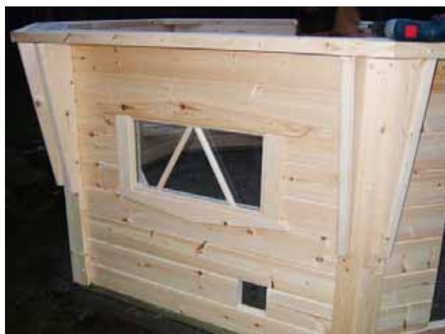
23. Install the windows and fasten the molding.
