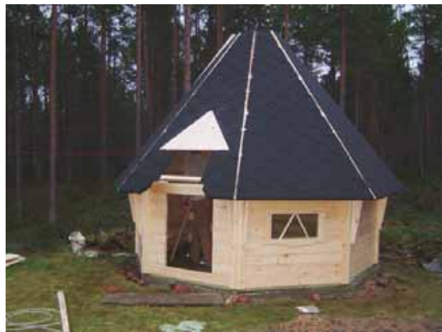
29. Put all of the roof elements in place.
